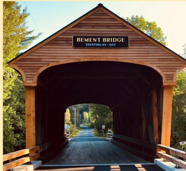
Bement Bridge renovation completed June 2021
