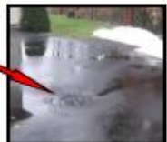
Custom poured concrete structure with outlet pipe cast near bottom. Pipe extend to daylight outlet. Structure carries away storm water from middle of paved driveway where ice dams had caused it to collect
