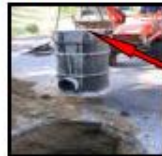
Custom poured concrete structure with outlet pipe cast near bottom. Pipe extend to daylight outlet. Structure carries away storm water from middle of paved driveway where ice dams had caused it to collect
