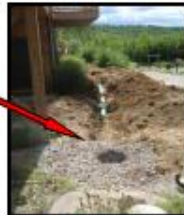
Light duty catch basin with 6" outflow pipe to daylight
