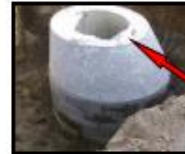
Industrial strength for under commercial parking lot across from Daily Sun. Porous concrete structure surrounded by stone
