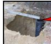
18" plastic pipe provides a base for cast iron grate and a reservoir and distribution area for water to soak away through holes in the pipe. Filter fabric covers several yards of 1 1/2" drainage stone surrounding catch basin. Installed at edge of development road.
