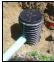
Light duty catch basin with 6" outflow pipe to daylight
