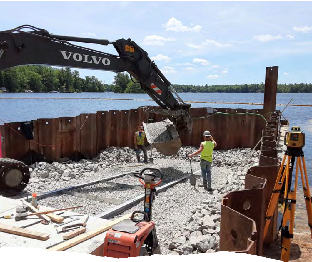
SETTING RAMP ANCHOR AND RAILS IN PLACE
