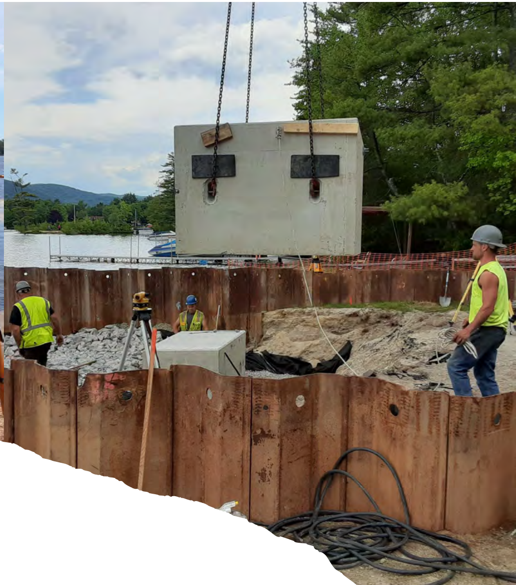
SETTING RAMP ANCHOR AND RAILS IN PLACE
