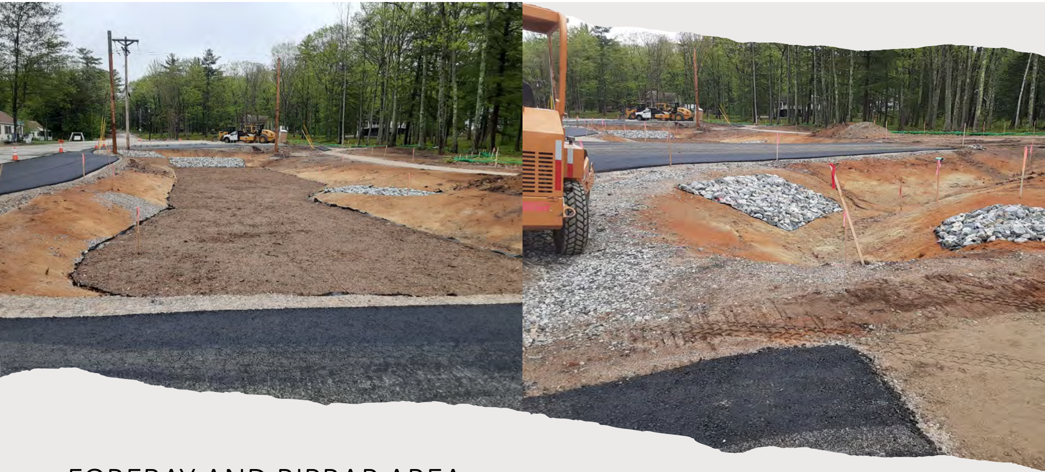
FOREBAY AND RIPRAP AREA CONSTRUCTION
