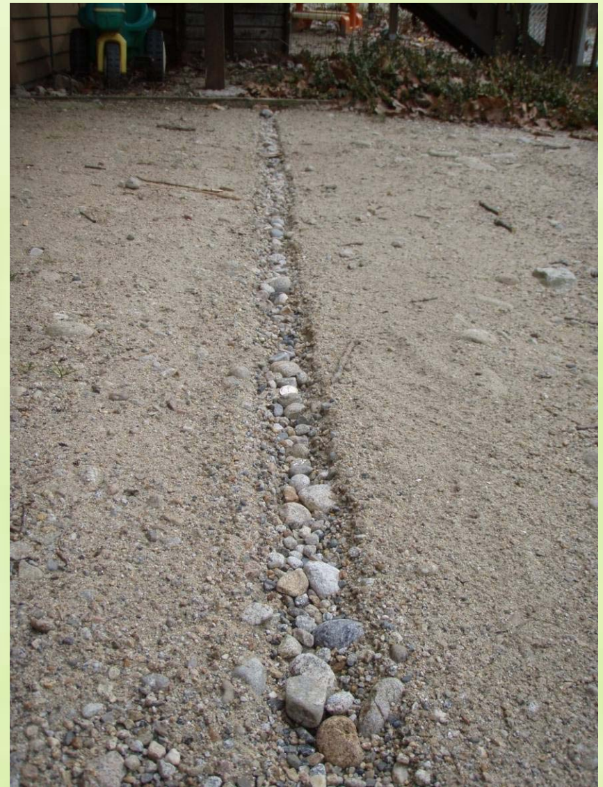
Concentrated roof runoff and resulting sediment displacement
