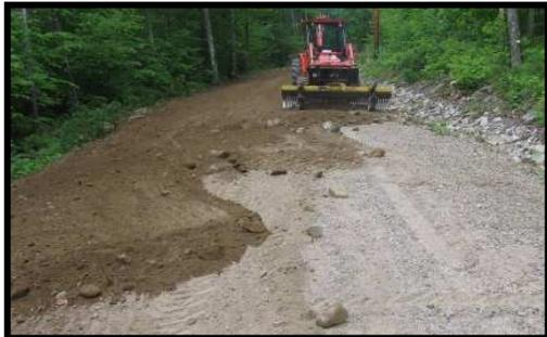
Cutting too deep into the surface of many roads can dig up rocks from the base that might be too big to reincorporate in the crown of the road and would better off left in place rather than lost to the side of the road during cleanup
