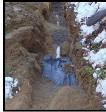
**Installation of an underdrain on the uphill side of a private driveway to remove groundwater**
