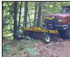
**Drive downhill and turn toward the ditch, penetrating the berm and forming a water turnout**
