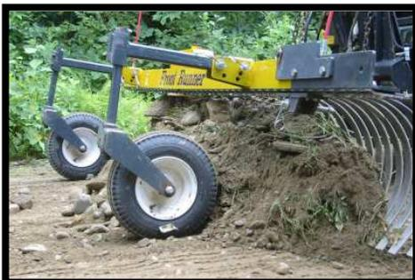
After material has been pulled to the center of the road and debris removed from it, the rule to follow is never to straddle the centerline with the wheels of the vehicle to which the rake or blade is attached unless it can be adjusted in the same manner as a road grader. Violating this rule generally means cutting down the centerline crown while attempting to clean and smooth the surface.
