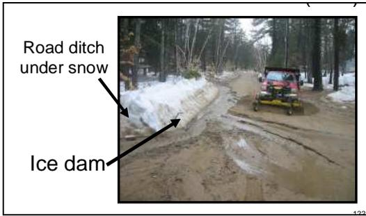
**This development road washed out because water could not reach the ditch at left and required some emergency repair.**
