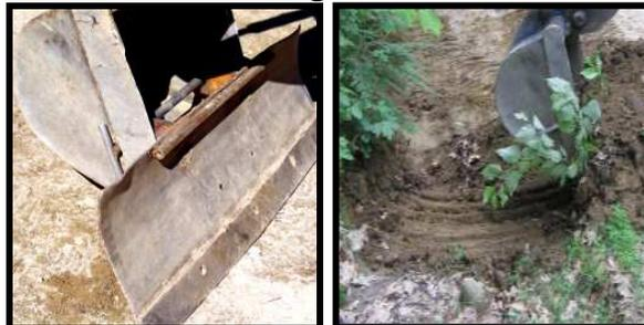
**Switch to backhoe where ditch becomes more defined and deeper than the road shoulder. This backhoe bucket is equipped with a 4' wide blade that pins onto the bucket providing extra width and eliminating teeth marks, leaving the bottom of the ditch smooth.**
