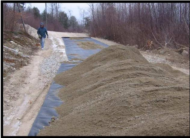
Geotextiles keep the gravel on top from being pushed down into the soil underneath, compensating for a poor road base
