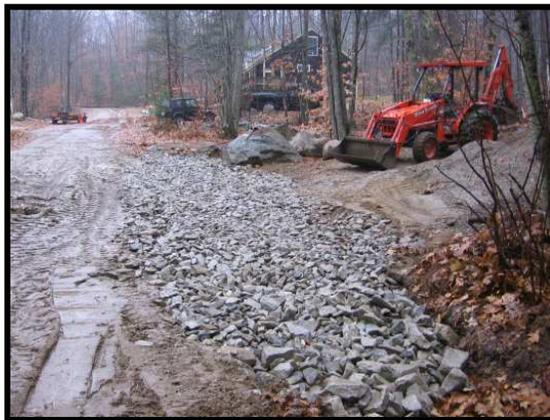
Another dip at the side of a development road across a private driveway with a substantial springtime flow across it, before surface gravel was added. Note the largest stone is 6" with 3" and 1.5" stone filling the voids.  $\frac{3}{4}$ " gravel forms the final surface, filling remaining voids, so that the stone disappears and the surface is smooth and firm to walk and drive on, but running water cannot erode the stone.
