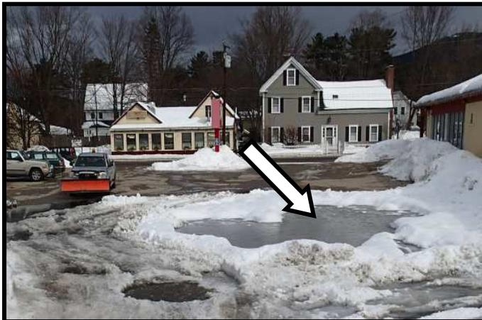
The catch basin in the middle of this large parking lot has been plugged for years making the lot extremely difficult to maintain in winter as well as a challenge for those who have to drive through it when there is over a foot of standing water and ice chunks. Arrow points to the submerged catch basin in late March 2014.
