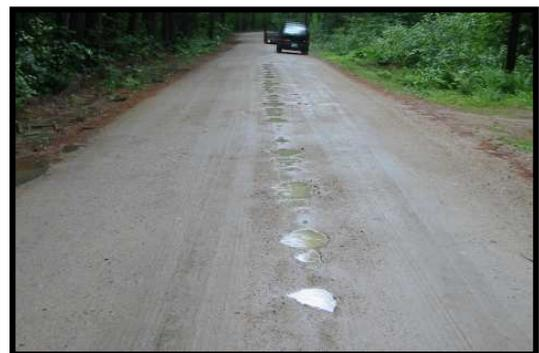
**Potholes down the middle where the road is the flattest and where most drivers put their left wheels**
