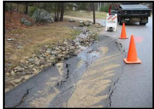
These two photos show water damages to the edges of paved roads due to poor ditch stabilization at the side.
