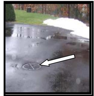
Other times it is necessary to collect stormwater runoff from a roof or other area and send it harmlessly away through an underground pipe rather than have it add to other roadway rainfall.
