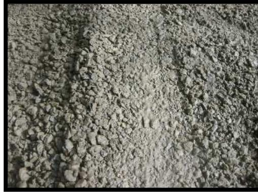
Here ¾" stone is being added and worked in with the grader/rake to form a strong surface that resists rutting
