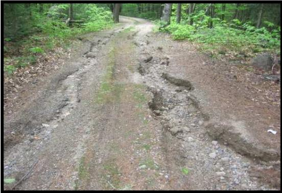
These washouts are the result of lack of maintenance in time to smooth out the wheel tracks caused by everyone driving in the same location (double ruts). Heavy rains followed the tracks even though this is only a gradual slope.
