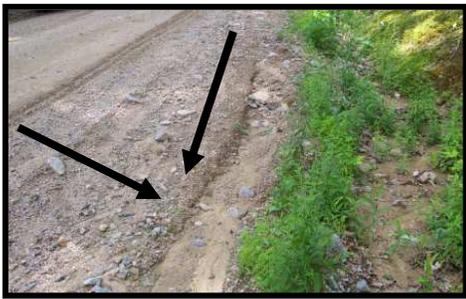
**Permanent grader berm left during years of poor grading practices. Note the ditch at right, but water is forced to traveling IN the road. (arrows)**
