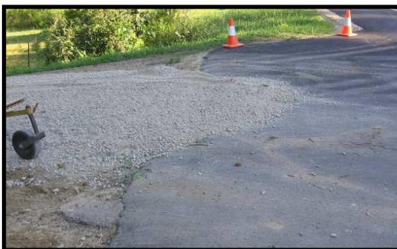
Though having some gravel cover the asphalt in a V or "hip roof" configuration may look like a mistake, it is an effective technique to reduce potholes at the gravel to pavement transition.
