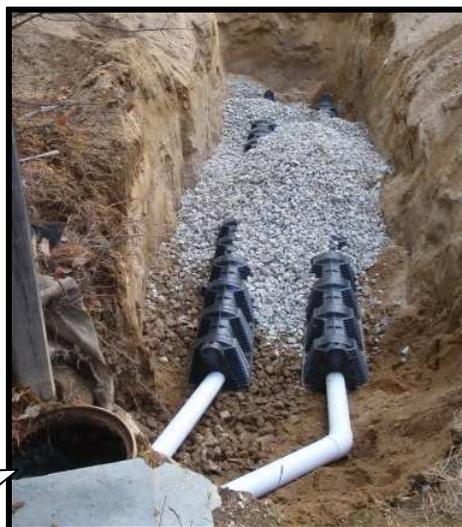
Lower two photos show a low cost addition to an existing catch basin constructed in very porous river gravel. The trench was excavated, the rocks raked out of the excavated material and placed back in the trench with two distribution pipes run out of the catch basin on top of the rocks which are then covered with filter fabric and backfilled.
