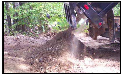
**Adding “ditch mix” that consists of several sizes of crushed stone from several inches down to small stone and some fines to hold it together. “Tailings” from a gravel producer can work very well for this purpose. Otherwise, mix several sizes of stone together, sometimes as large as 6” depending on the application. This particular crossing was lined with tailings.**
