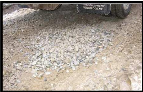
Small pockets of mud or mudholes can usually be repaired with the addition of crushed stone in the same manner as deep muddy roads (11.1.2). If the source of the problem is an active spring, however, it is preferable to install a subsurface drain to remove the water from the roadbed
