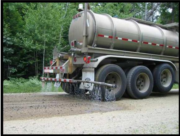
Calcium chloride can also be applied as a 35% liquid when mixed with water by a delivery truck with a built-in distribution system. For a first time application the rate is .3 gallons per square yard with follow up applications of .2 gallons. Many towns now do this regularly and report significant savings on road maintenance.
