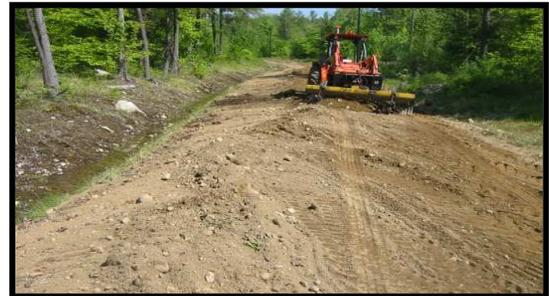
**For this driveway reconstruction, shoulders have been pulled in with a tractor to form a substantial "lift" in the middle of the road and grading has begun**
