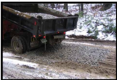
If a road turns to impassible mud in the spring, the only practical way to return it to service immediately is to add crushed stone (not gravel) to strengthen it. Use larger (1½" stone) until road firms up. It's generally cheaper and stronger than  $\frac{3}{4}$  stone. Stone is worked into the mud until the road is able to support passing loads. Though expensive, this scheme is very effective for emergency repairs.
