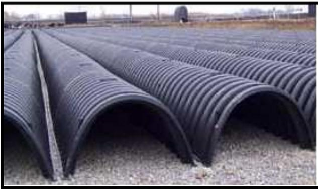
This is an example of a large scale storm water storage and infiltration system being installed under a municipal or a large mall parking lot to return stormwater to the ground
