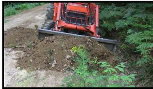
**Using a loader front bucket to clear ditch of debris and remove grader berm**
