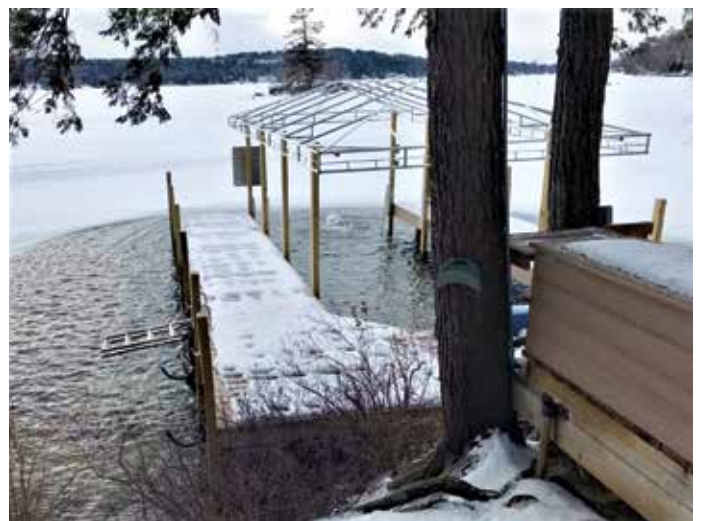
This is an example of how to de-ice around a dock without creating an open water area that extends beyond the property. (Photo Credit: Watermark Marine Systems, LLC)
