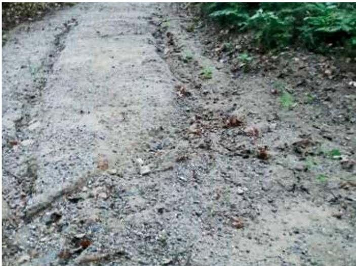
*If your gravel road or driveway has fully developed ruts like this, surface waters nearby are in danger of being polluted with silt and nutrient laden runoff water.*
