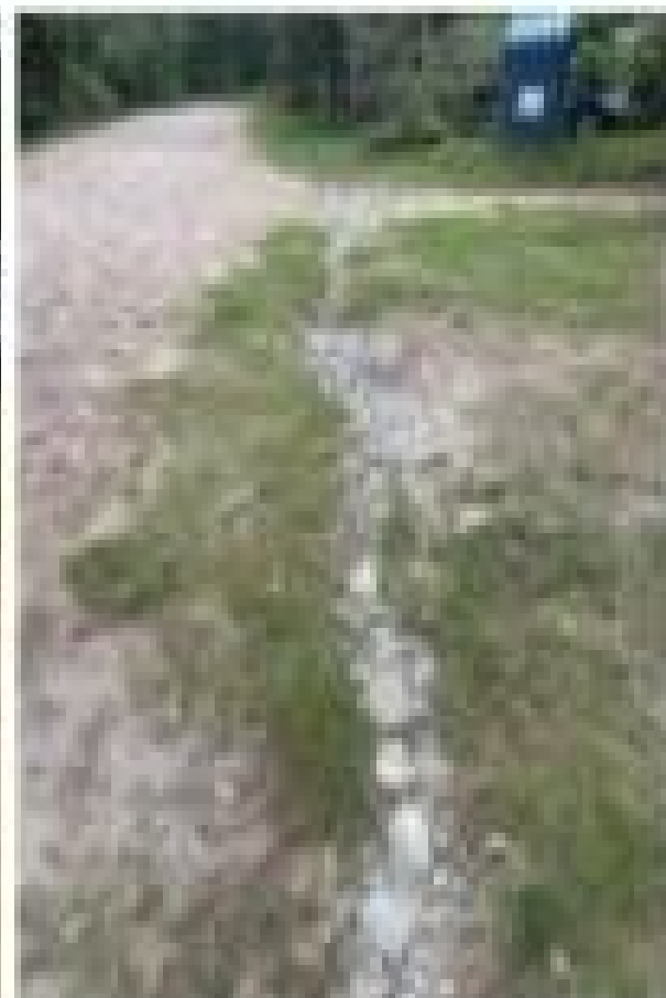
(Left) Steep grade leading directly to beach area/lake, (Right) eroded left side of road running off into gully.
