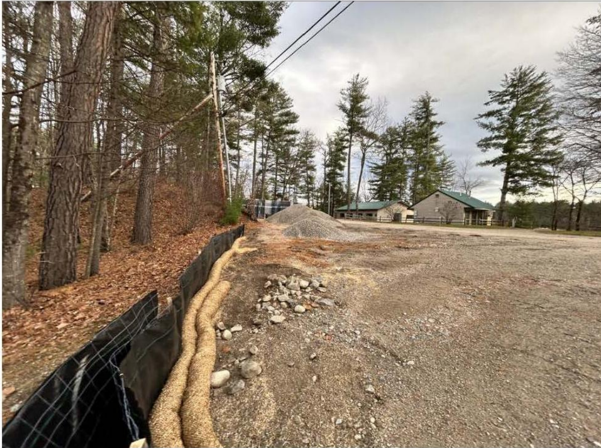
Figure 2: Erosion Control Installation
