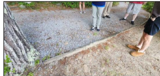
Figure 3. Example of lumber edging along a gravel road noted at another NH lake.
