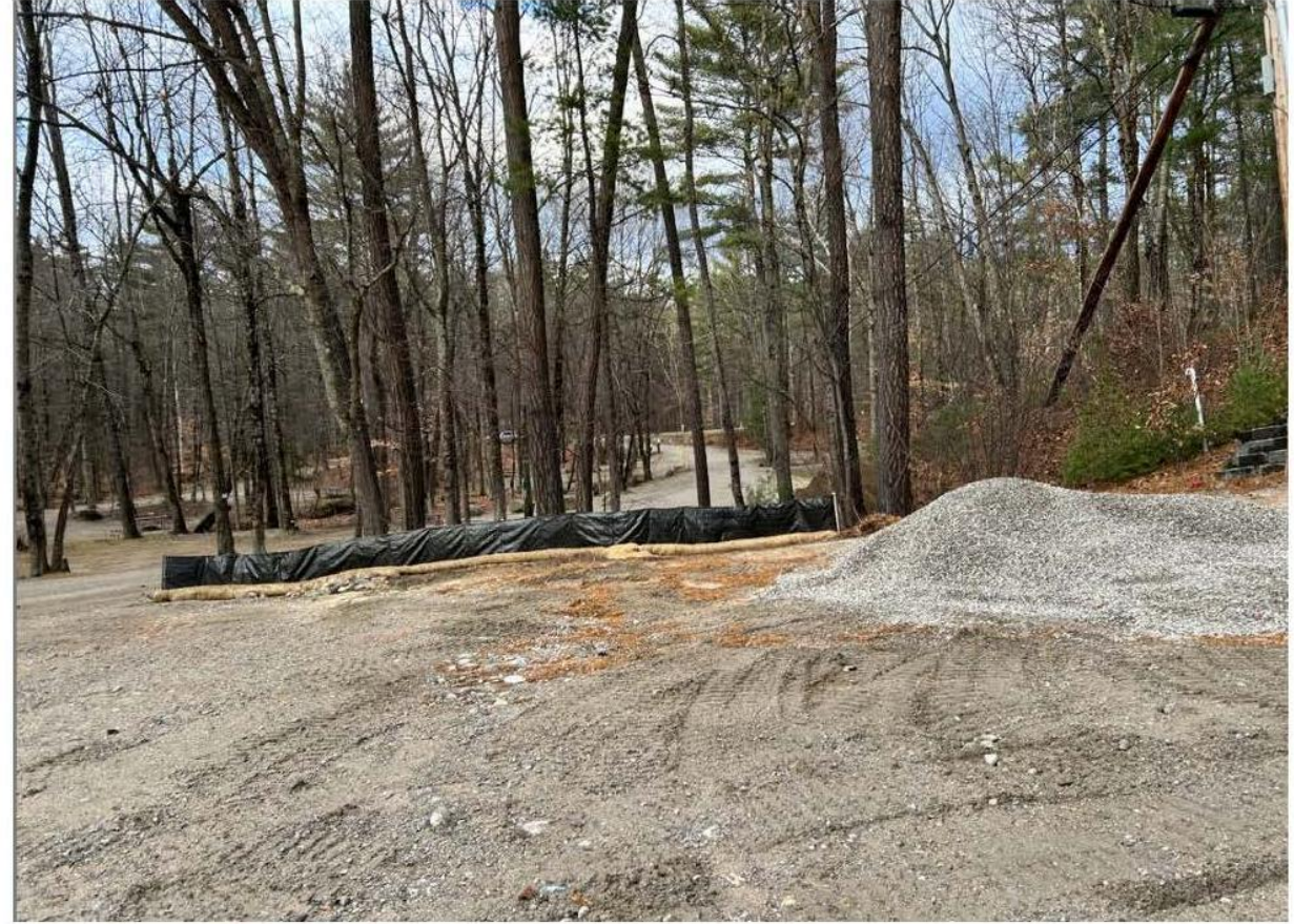
Figure 1: Erosion Control Installation
