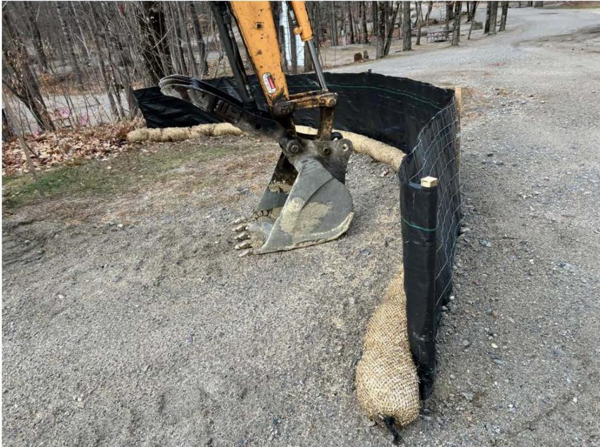
Figure 3: Erosion Control Installation
