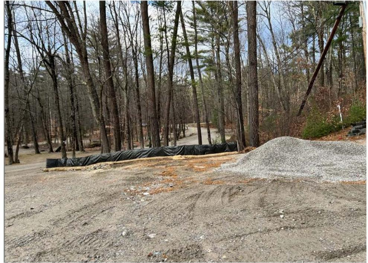
Figure 1: Erosion Control Installation
