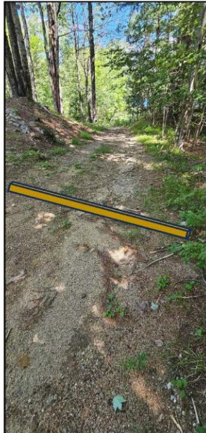
Figure 1. Water bars are set at an angle to the slope and designed to prevent runoff from traveling further down the slope.
