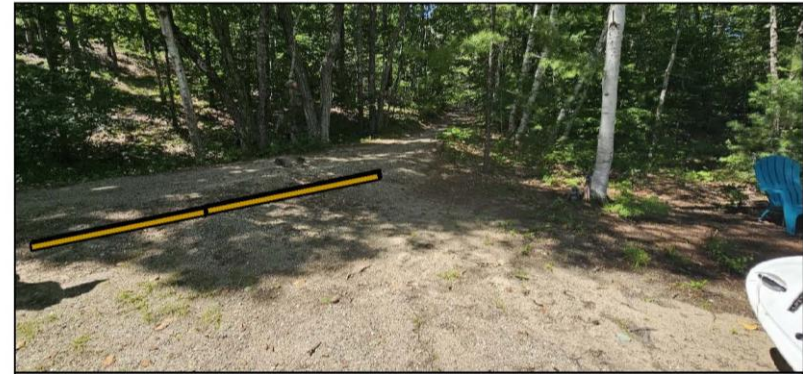
Figure 2. Install lumber edging to prevent road runoff from spilling into access area and into the pond.
